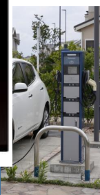
Two EVs are reserved. In case of an emergency, the V2H system supplies electricity to the assembly room, etc.
